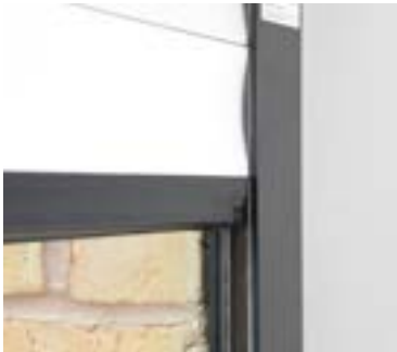
Heavy duty extruded aluminium guides secure the door at the sides.
